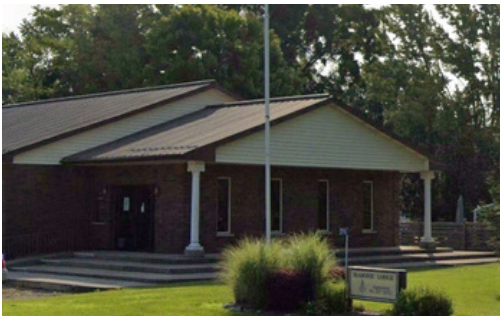
Wardsville Masonic Hall
